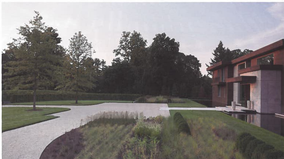
Views of the front yard (above) depict the level of disturbance created by the architecture. The subterranean parking structure serves as the foundation for the 11,500 SF intensive green roof, which extends from the house to the center of the entry-court.
