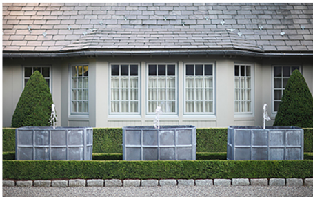
Lead planters, inspired from England, were converted to water features to add sound, movement and light to the front courtyard.
