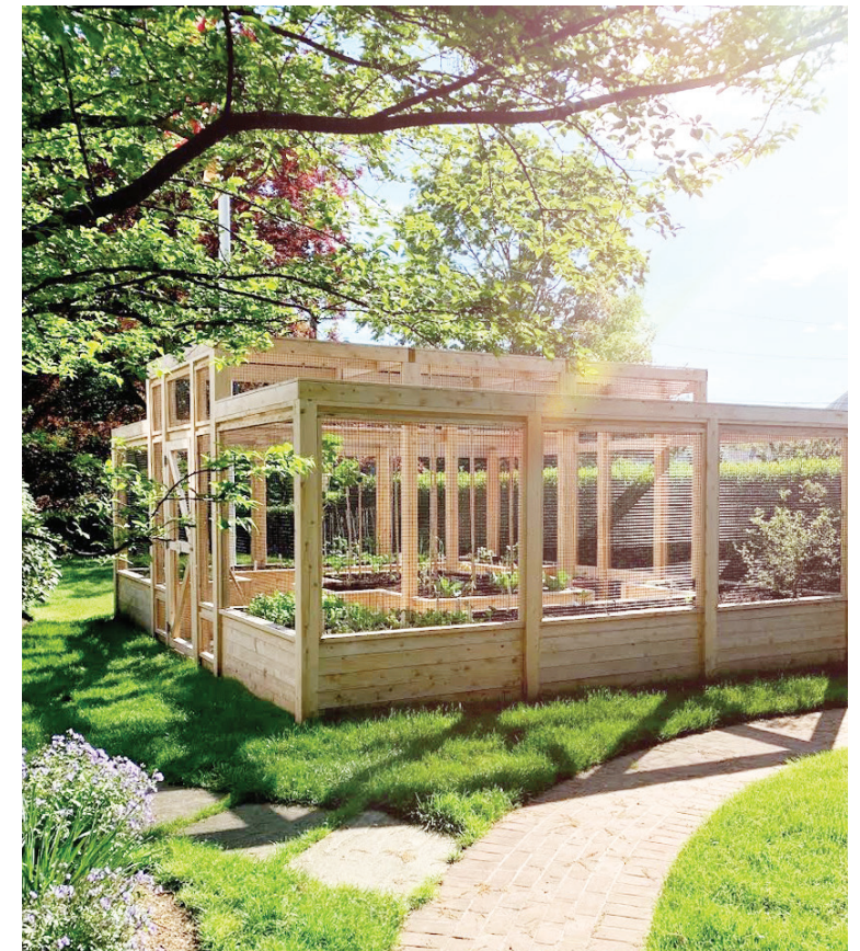
right: Architect Mark Finlay designed and Andrew Tyrrell built this custom garden structure out of white cedar and deer-resistant fencing.
